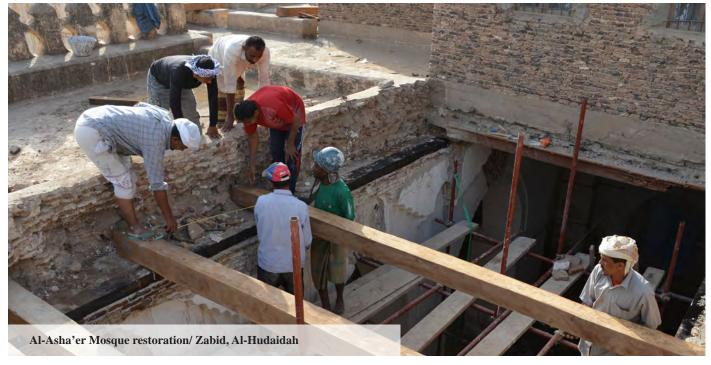
were made in the north part of the eastern pool to uncover the foundations and track damage caused by the water leakage over the past decades. Also, treatment, repair and replacement are being carried out for the wooden staircase of the minaret, which eroded due to termites, according to the same original traditional specifications.
