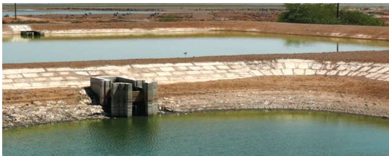
Wastewater management project (Al-Buraïqa, Aden)
