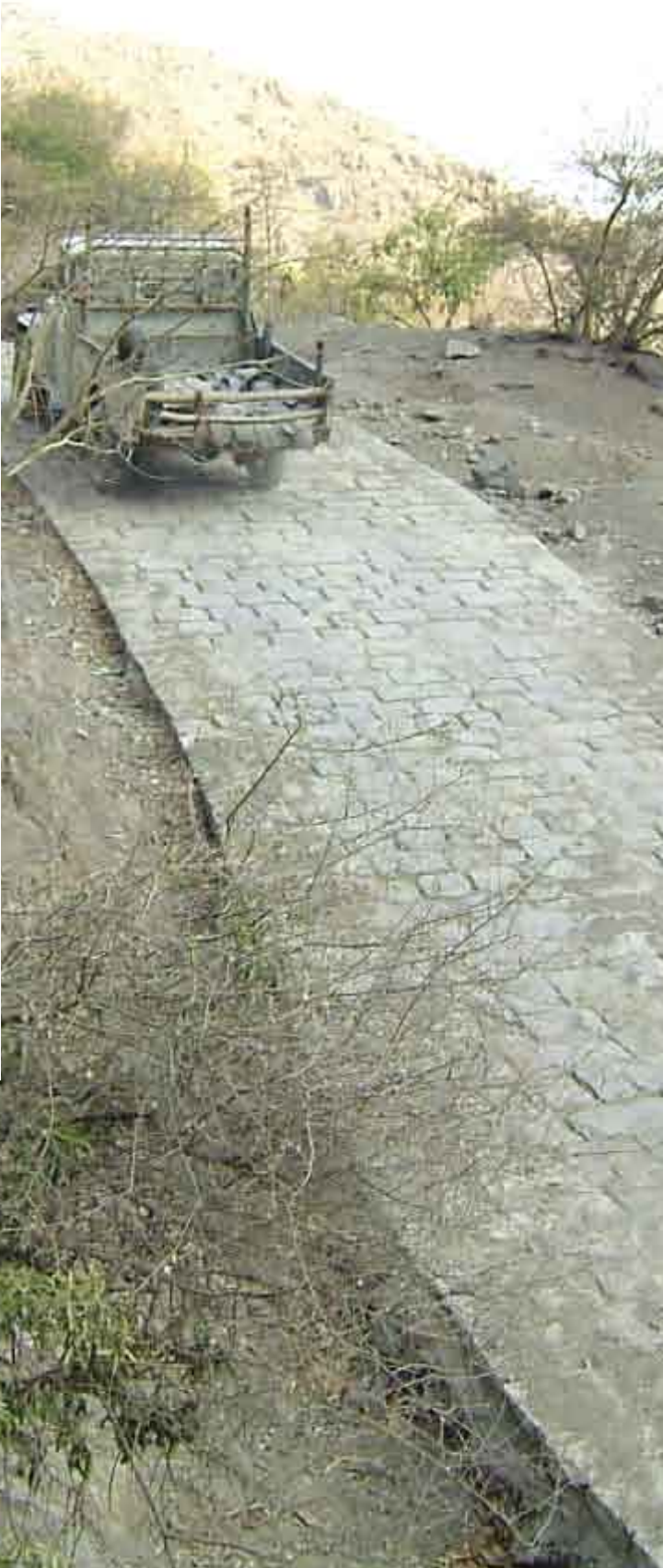
An SFD-supported rural road project (Bani Hat, Al-Odain, Ibb)
