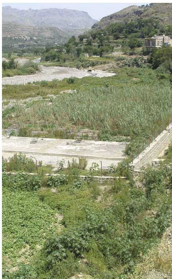
Wastewater management project (Al-Saddab, Ibb)
