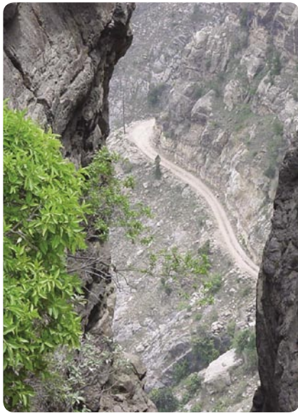
SFD-supported rural road in Al-Maqatera, Lahj
