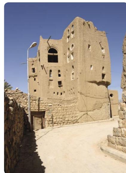
Street paving increases access to cities of historical value, as here in the old city of Amran
