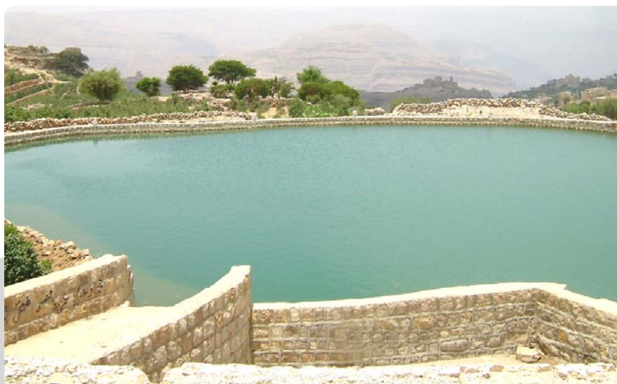
SFD-supported rainwater harvesting projects give communities sustainable sources of water (Al-Sawdah, Amran)
