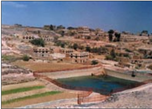
Cisterns for rainwater harvesting—a major SFD's activity aiming at providing water to rural communities
