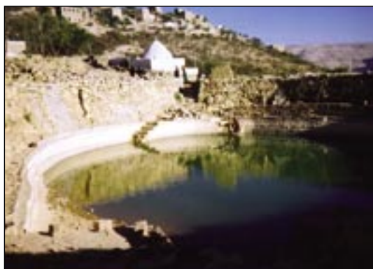
Traditional water collection is extensively focused on—a cistern in Marhaba, Dhibain, Amran governorate
