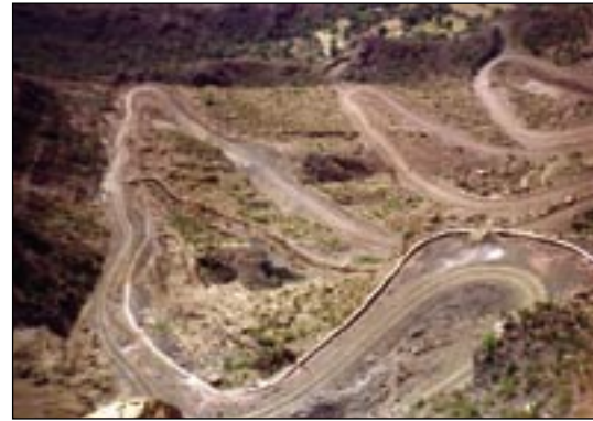
Rural roads are constructed based on remoteness, poverty and feasibility of the roads
